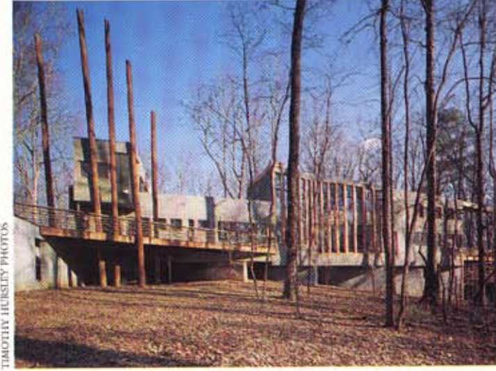
House Chmar Atlanta, Georgia Scogin Elam and Bray Architects
