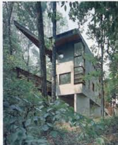
Chmar House, Atlanta (1989). The wooden and glazed private house was placed in a clearing of dense woods on the exact spot of a fallen tree. Bedroom terrace projects into the wilderness.
