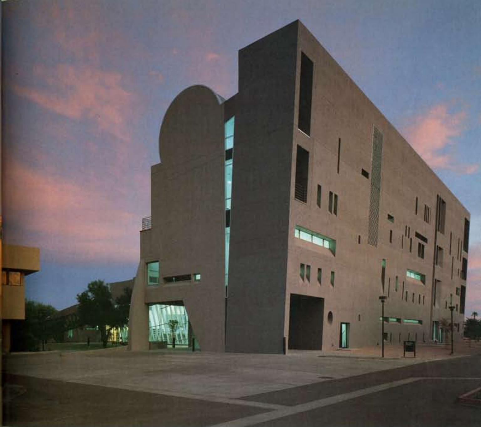
Desert conditions: the open, north side (opposite) contrasts with the closed, southern facade, protecting the interior from the sun.
