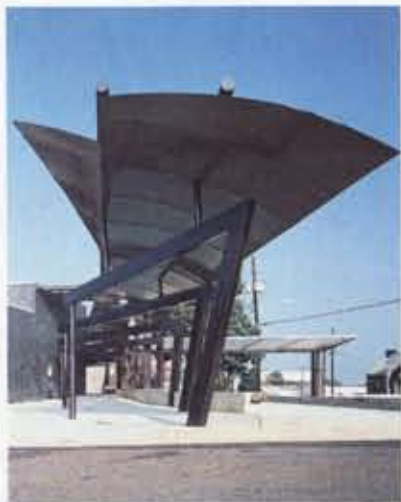
Buckhead Library, Atlanta (1989). One of two libraries by Scogin Elam & Bray that bring powerful architectural forms to a wasteland of drive-thrus and shopping malls.
