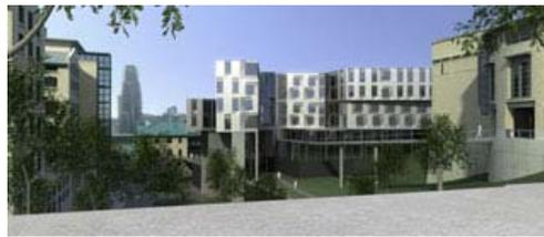
The Gates Center as seen from the Cut. The exterior, or skin, of the structure is still in question, however, architect Mack Scogin proposes that the building's exterior be 52% solid zinc or slate and 48% glass windows.
