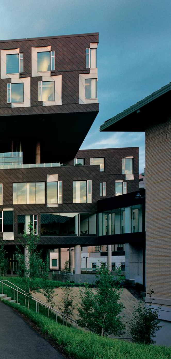
The sixth and seventh floors of the Gates Center (above right) are glass-enclosed and offset from the other floor plates. This glass volume is filled mainly with open project space and a collaborative commons, as well as conference rooms and select faculty offices. The glazing continues on the façades lining the courtyard spaces between the two buildings, creating a visual connection between them.
