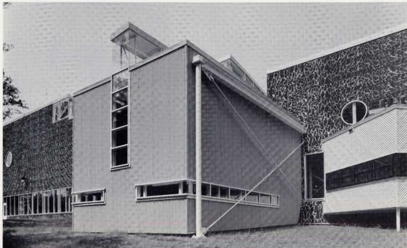
13, 14. Views of east elevation
