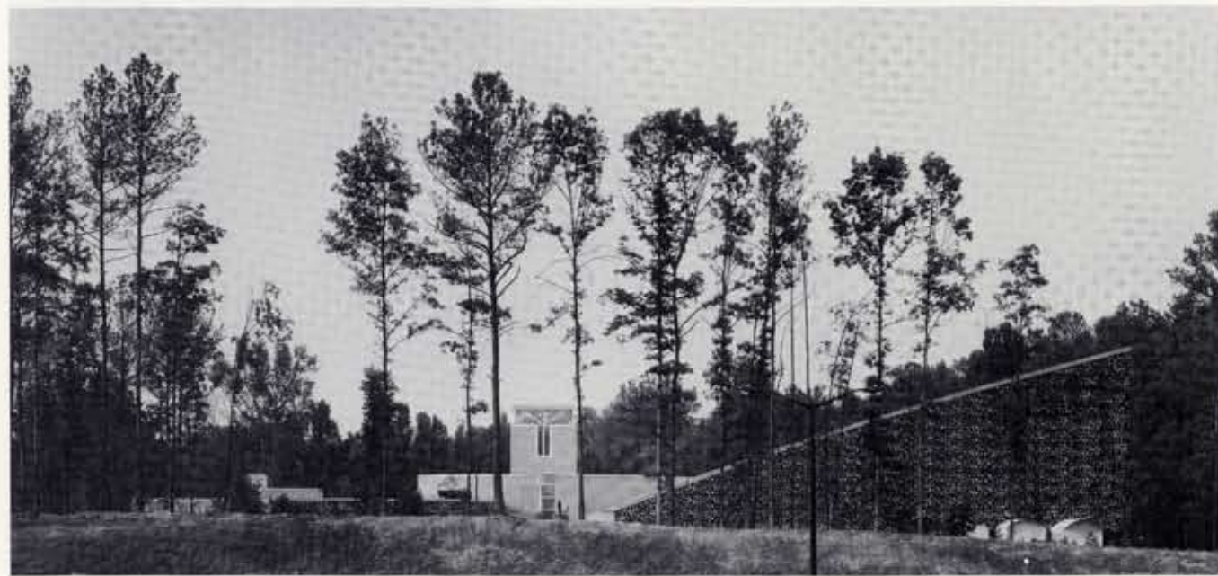
16-19. Views of south elevation
