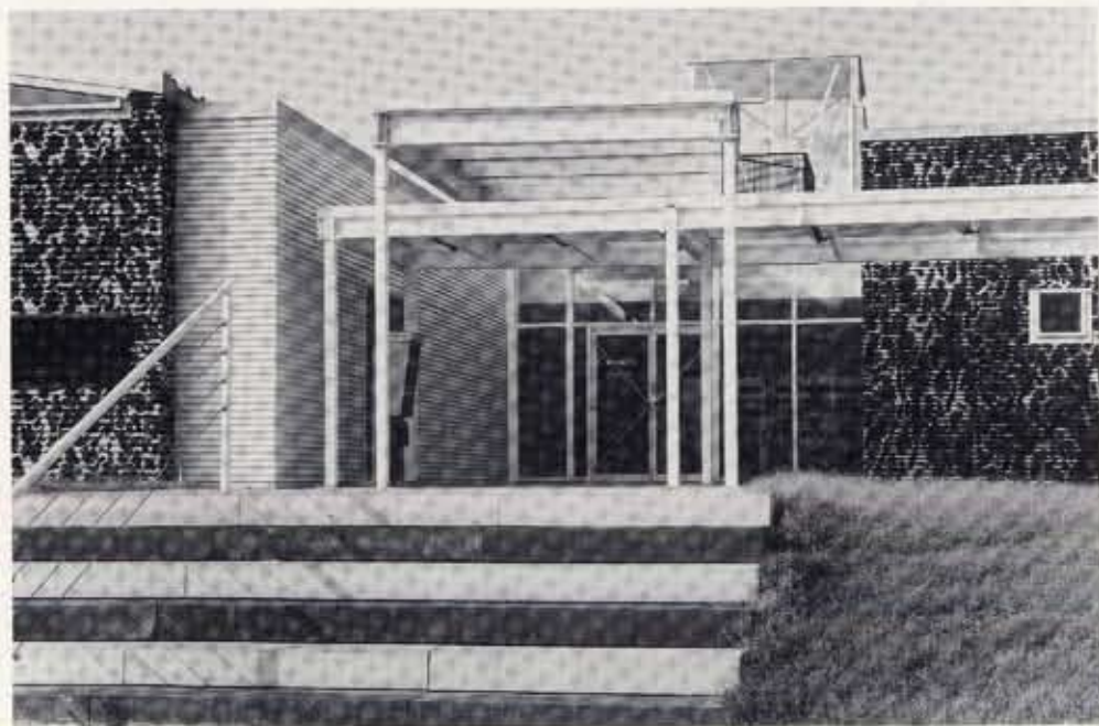
7-10. Views of north elevation
