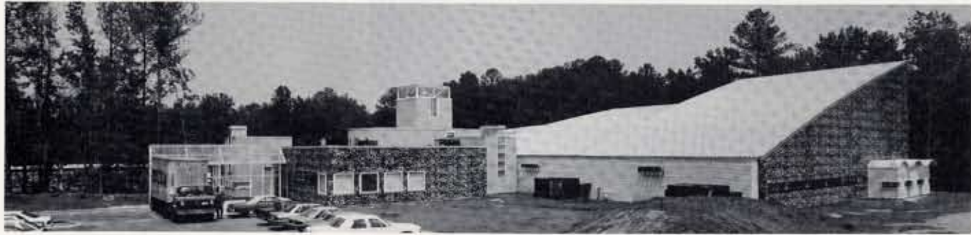
21-23. Views of west elevation
