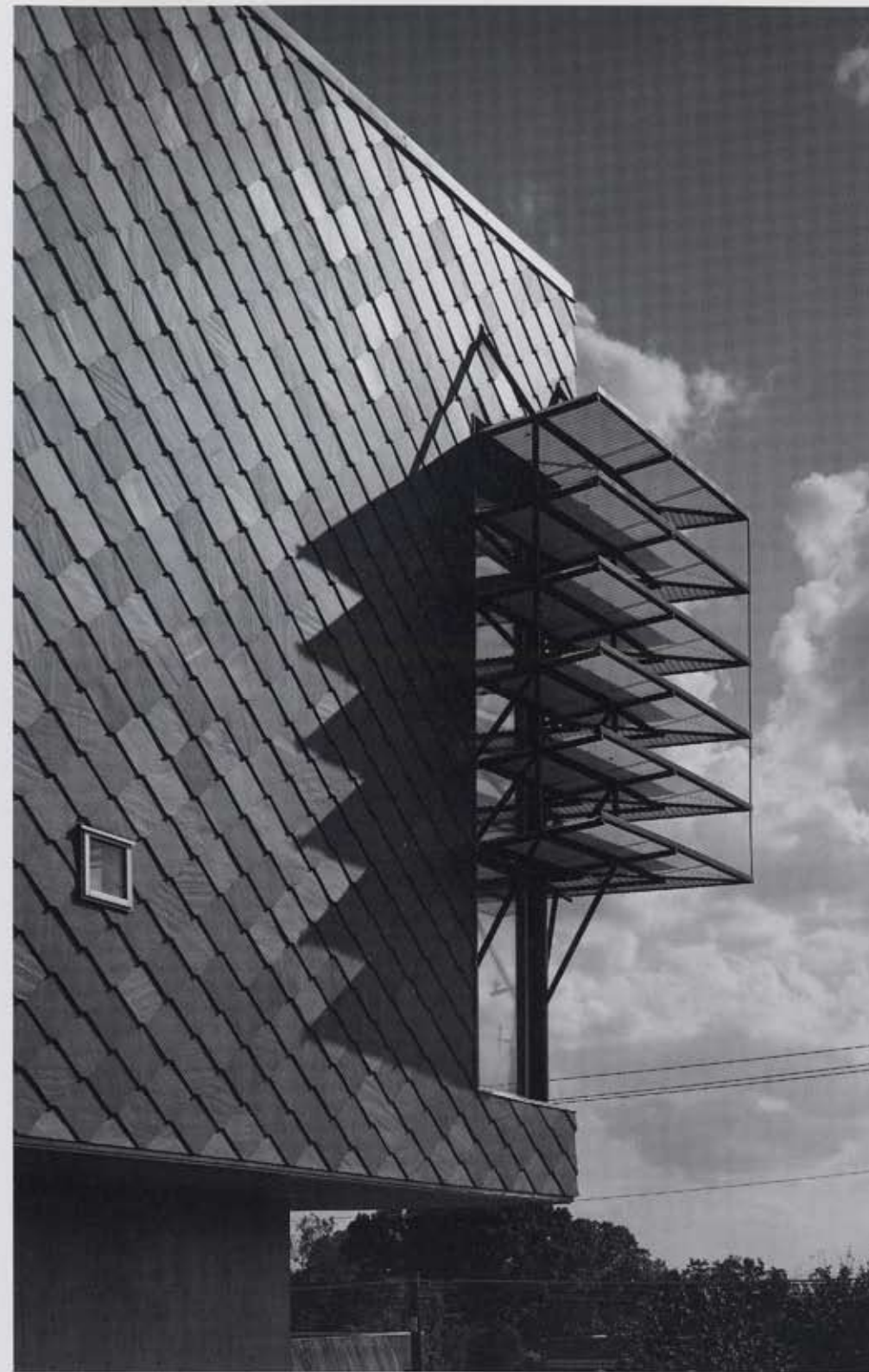
Southwest end 南西端部
