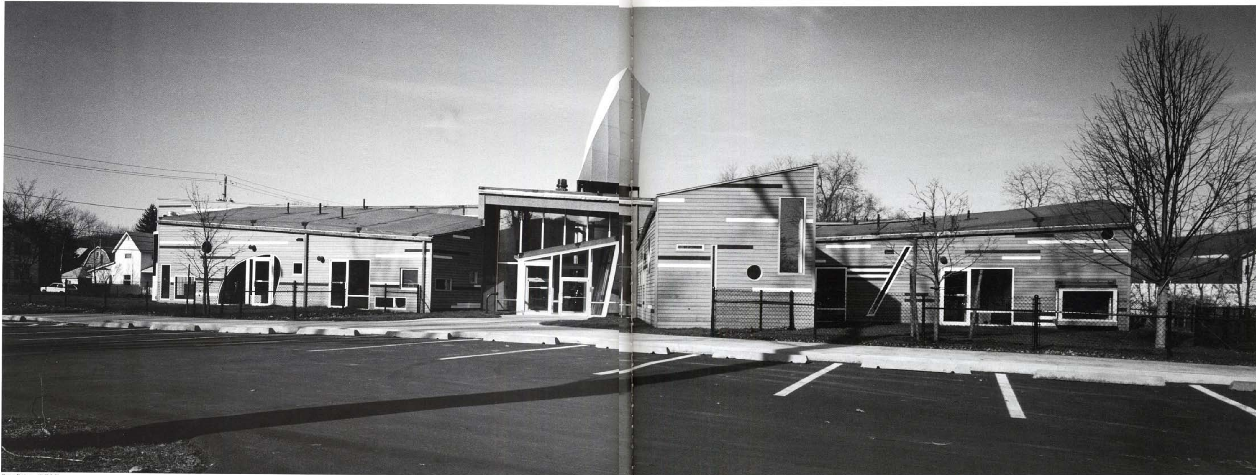
Overall view 正面全景
