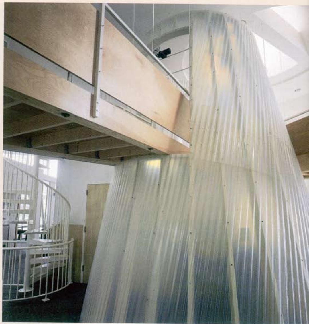
CORNING CHILD DEVELOPMENT CENTER CORNING, NEW YORK SCOGIN ELAM AND BRAY ARCHITECTS
