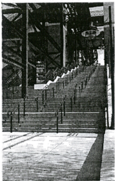
One of two grand staircases at the new Olympic Stadium, which will become the Atlanta Braves' home.
