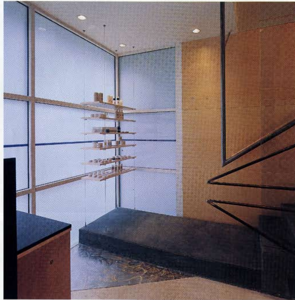
A skeletal metal system outlines the stair rail with raw structure, and etched acrylic and plywood panels line opposing walls (right). The entrance to the spa through the salon (top) leads to the translucent reception area (above).
