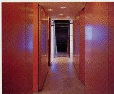
Plywood doors and walls in the ceramic-tiled-spa area are protected by phenolic resin-impregnated film (above and right). Stairs are sealed, pigmented concrete, exposed to the first-floor corridor (opposite).
