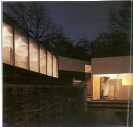
Above, a steel bridge connects the main house to a guest house and studio out back.
