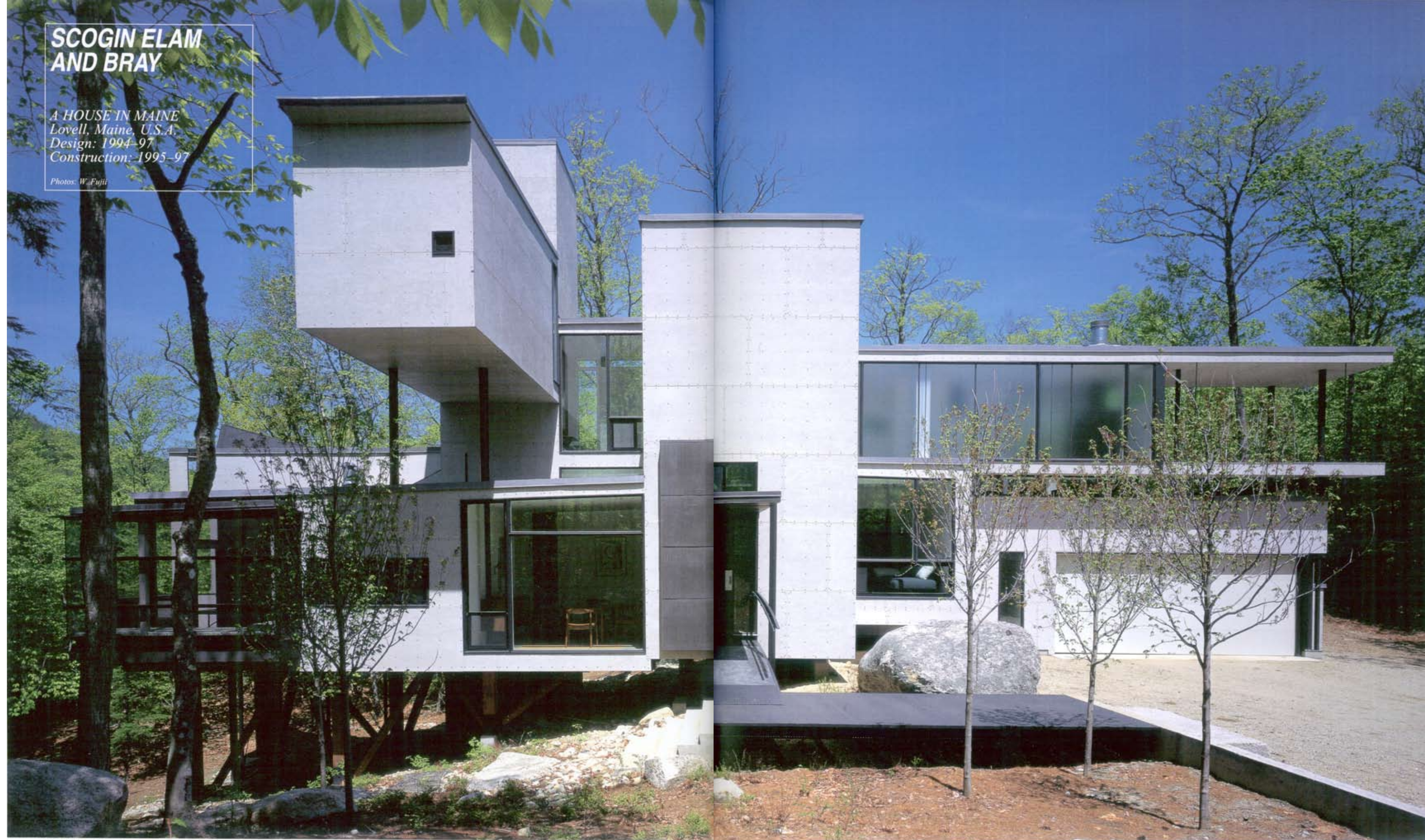
Overall view from east
