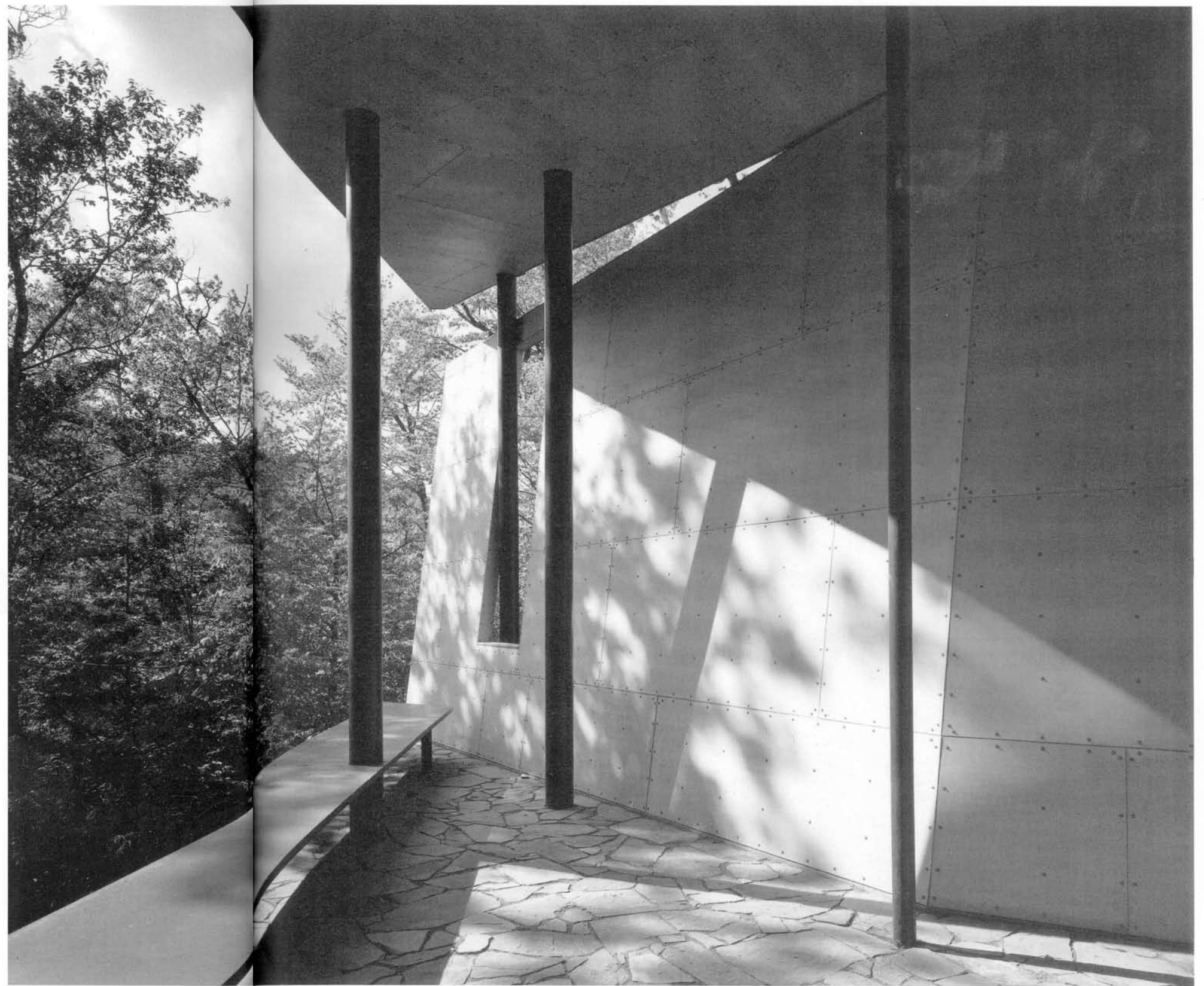
Deck on second floor
