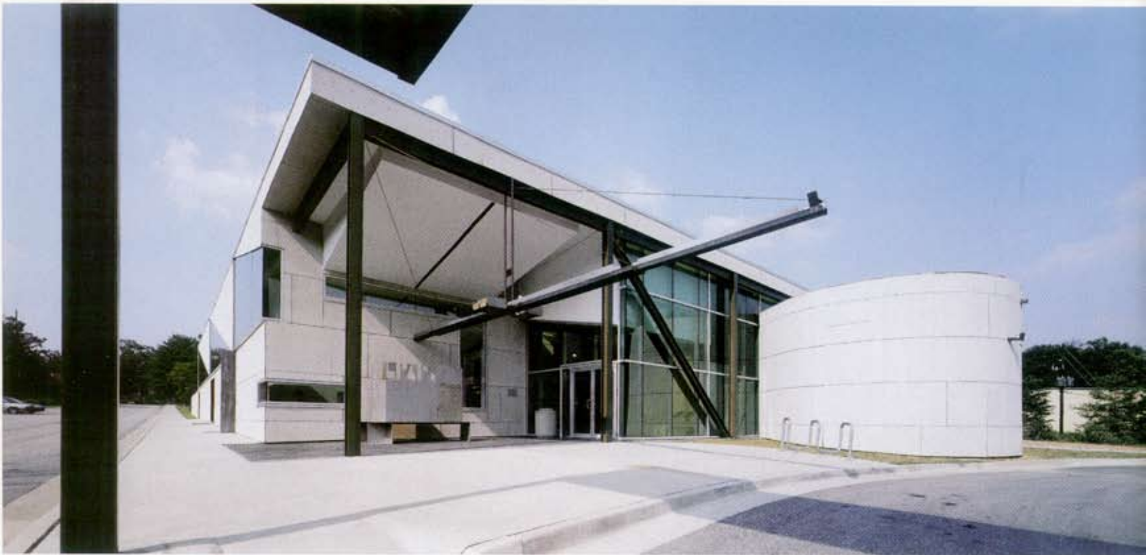
The architect exposed the library's steel frame on its south face (above). The curved form (at right) houses a meeting room that can be accessed through the lobby for after-hours events. The fiber-cement panel-clad lower half of the library's lean east side (below) extends to enclose a north-facing garden (facing page, below). The zigzag profile of the roof trusses (section, facing page, center) echoes in the scissor pattern of the clerestory windows on the west facade (facing page, above).
