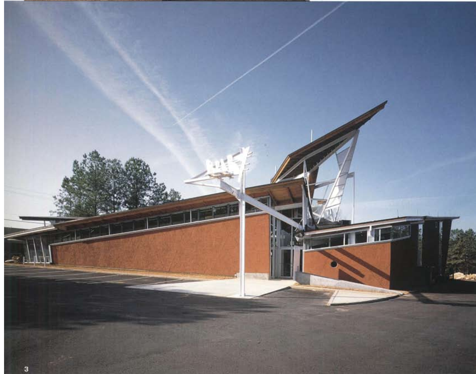
Carol Cobb Turner Branch Library, Morrow, Georgia: 1 Detail with children's handprints. Exterior walls are of glass and Georgia red clay-colored synthetic stucco; 2 Detail at children's area. Just outside is a small garden and reflecting ditch; 3 East elevation. The asymmetrical plan has a dividing breezeway/corridor with rooms off both sides, skewed up toward the bright blue sky and away from the flat, heat-filled, hostile site. Connections to other community buildings and neighborhoods, the points of the compass, and property lines all give form to the building. A vertical steel and glass tower serves as a negative center support, from which the mushroom-like roof emerges on a simple post-and-beam structure. Photo credit: Timothy Hursley
