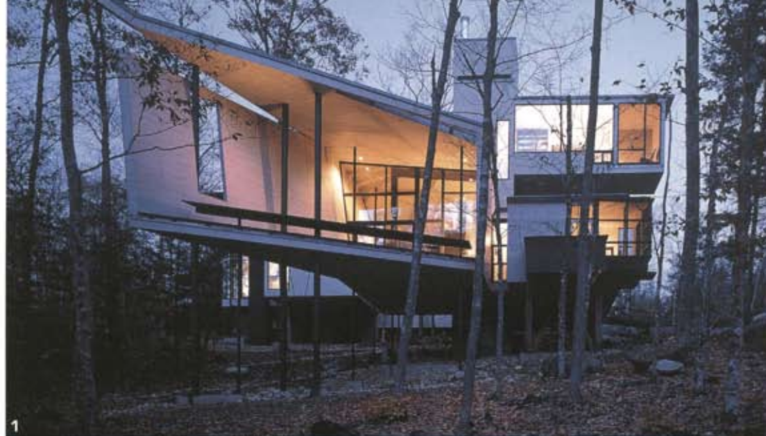
Nomentana Residence, Lovell, Maine: 1 Western elevation, showing forms added onto forms. Rooms are always in spatial and visual continuation, giving the impression of small "house-towns" that resist feelings of isolation in the rural Maine setting; 2 View from living room deck toward pond and mountains; 3 View of living room toward deck; 4 View of entry/library. Photo credit: Timothy Hursley
