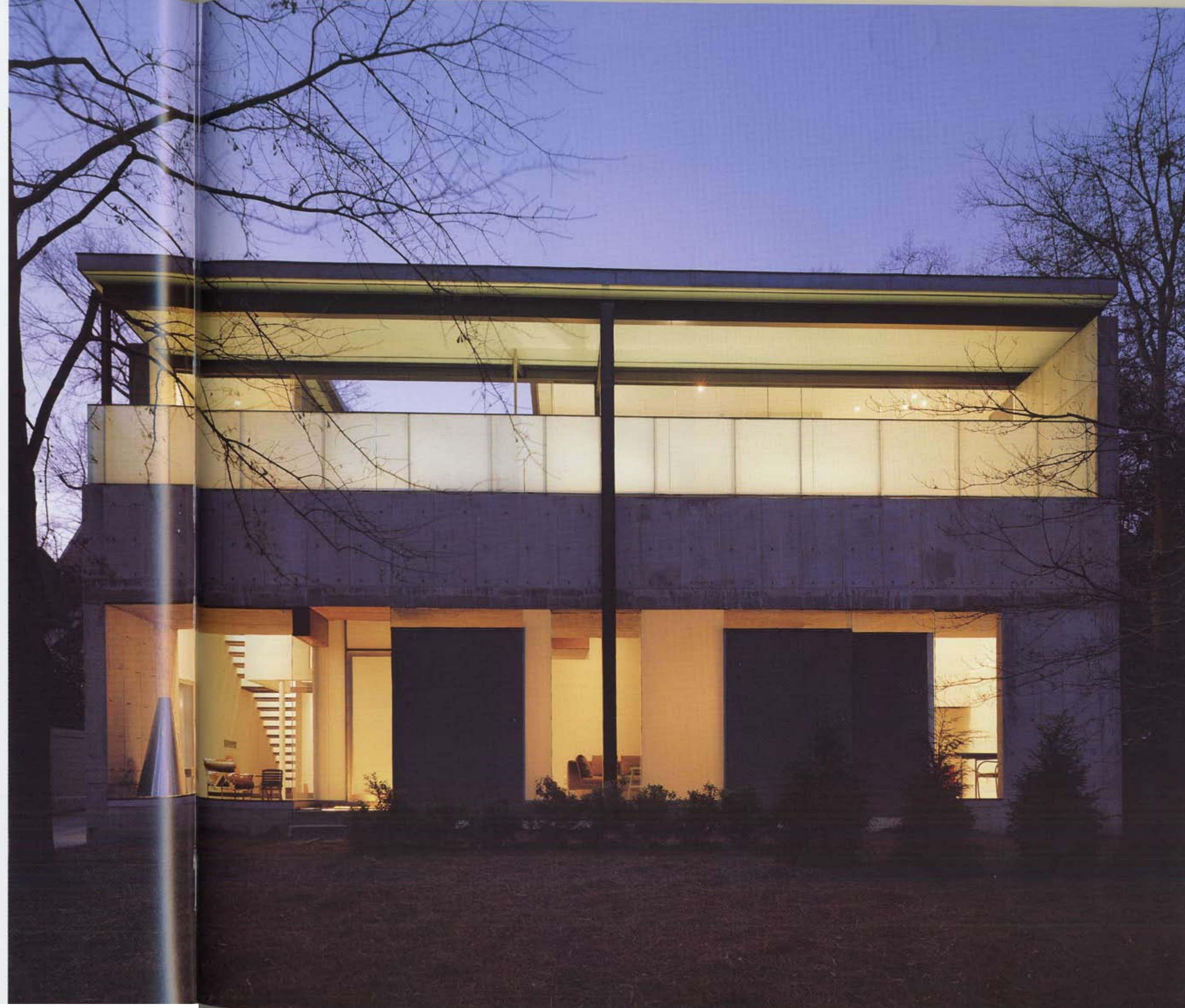
BELOW: Street façade BOTTOM: View of guest pavilion FACING PAGE: Street façade
