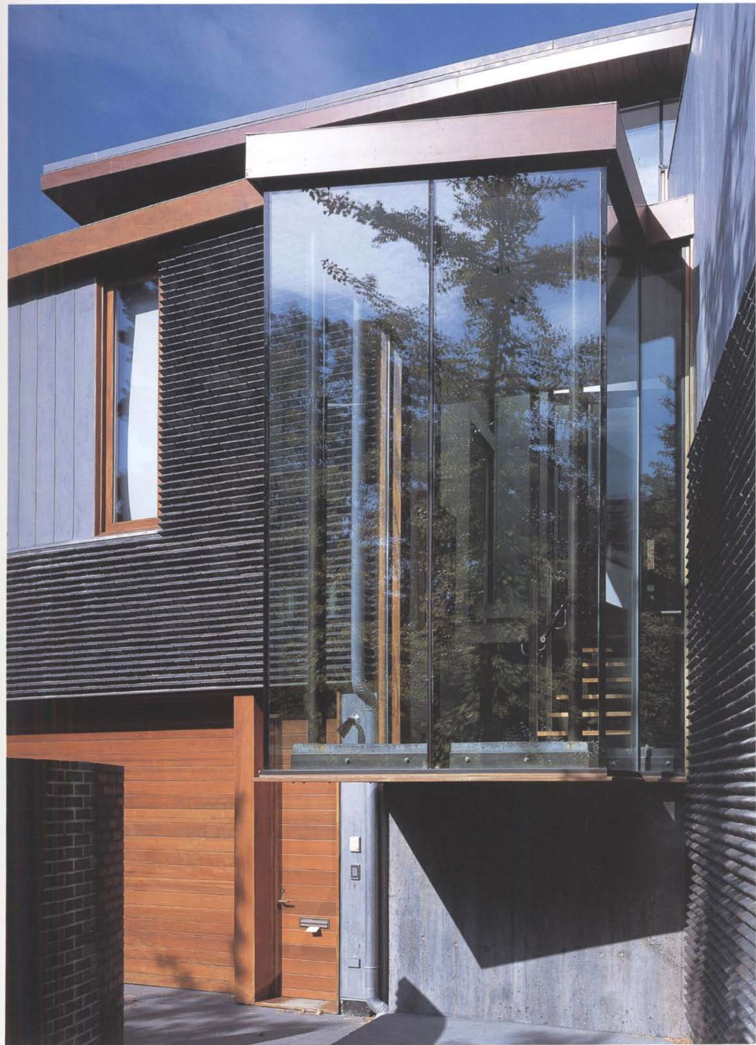
Glazed staircase: garage on left
