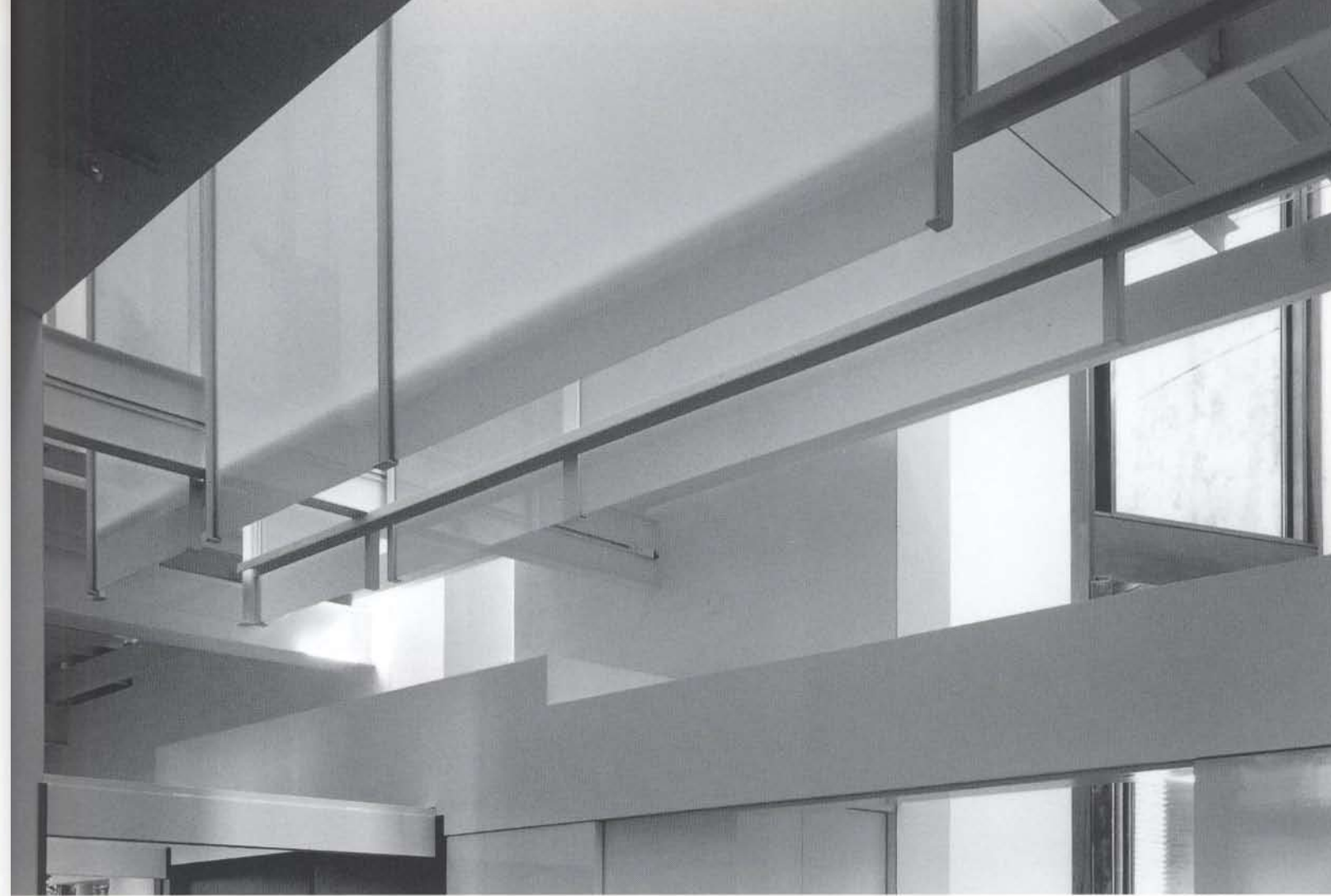
Detail of "light box"
