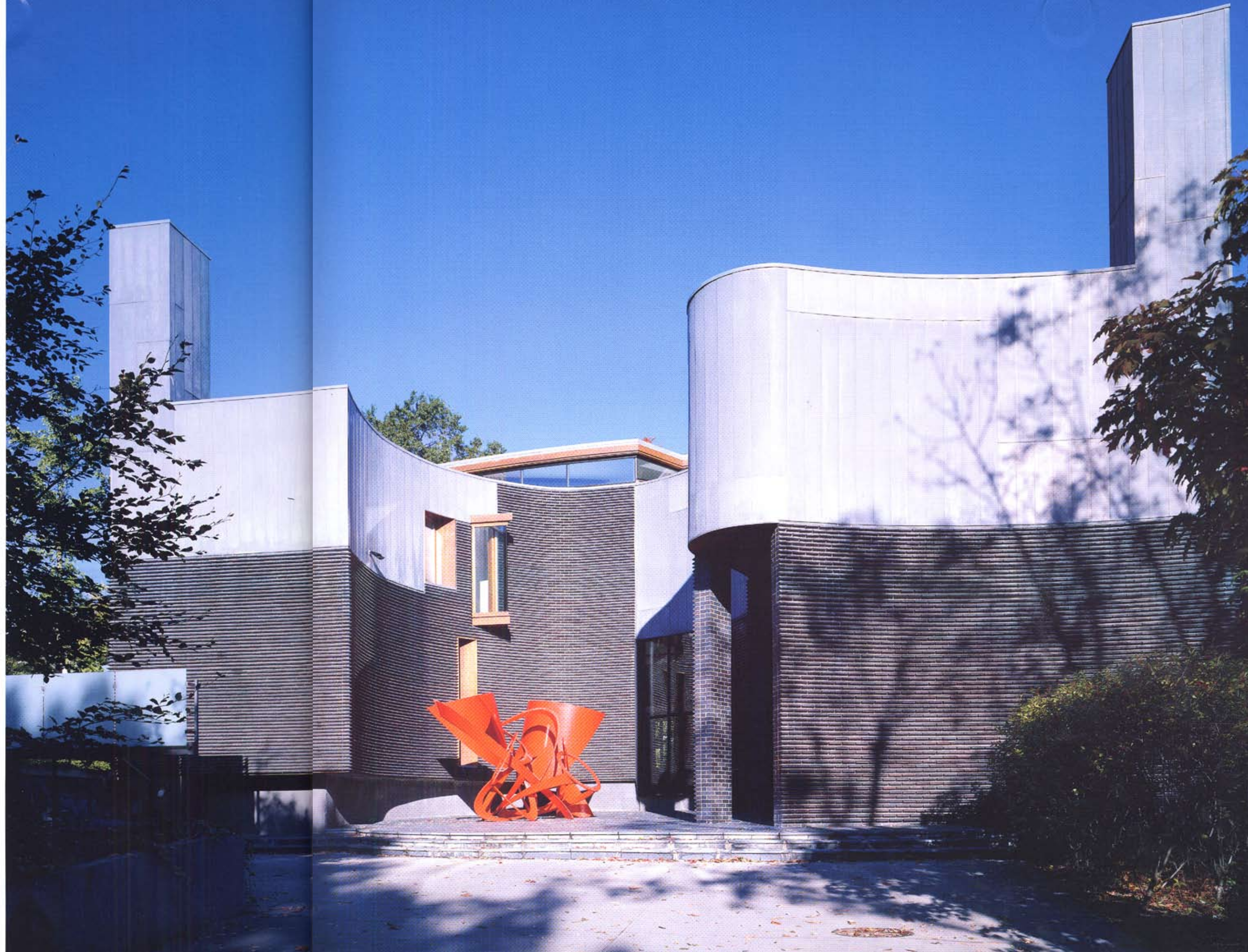
ABOVE: View of sculpture court from entry FACING PAGE: South elevation
