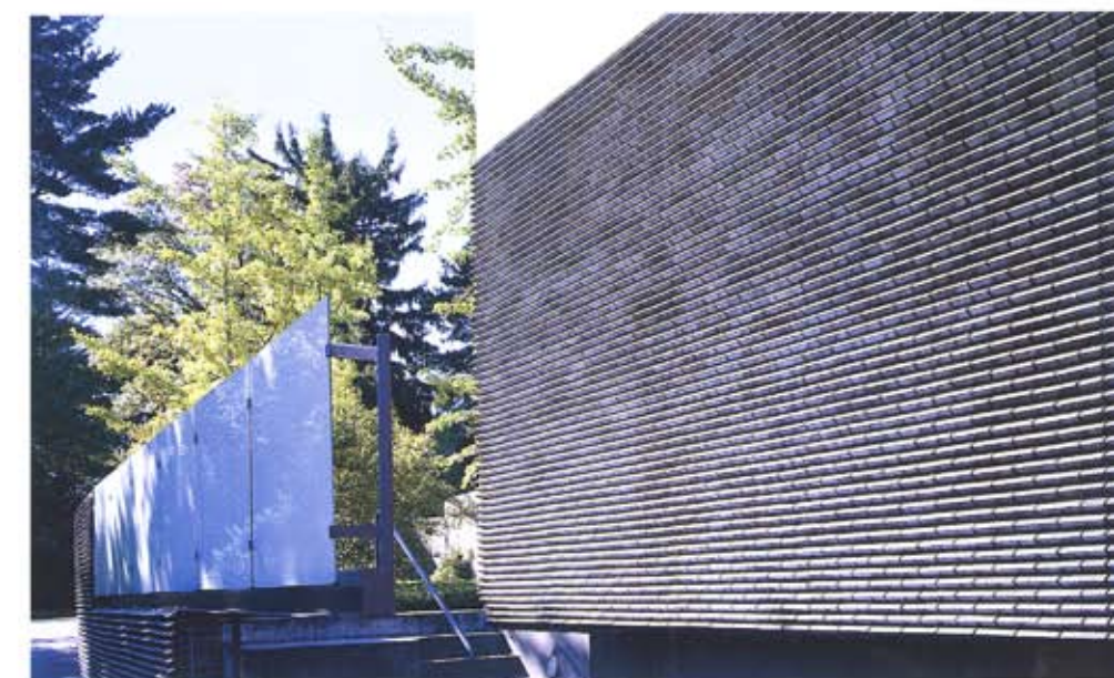
ABOVE: View from southwest LEFT: View toward stairs to walled garden FACING PAGE: Detail of lead-coated copper siding and custom Endicott brick siding
