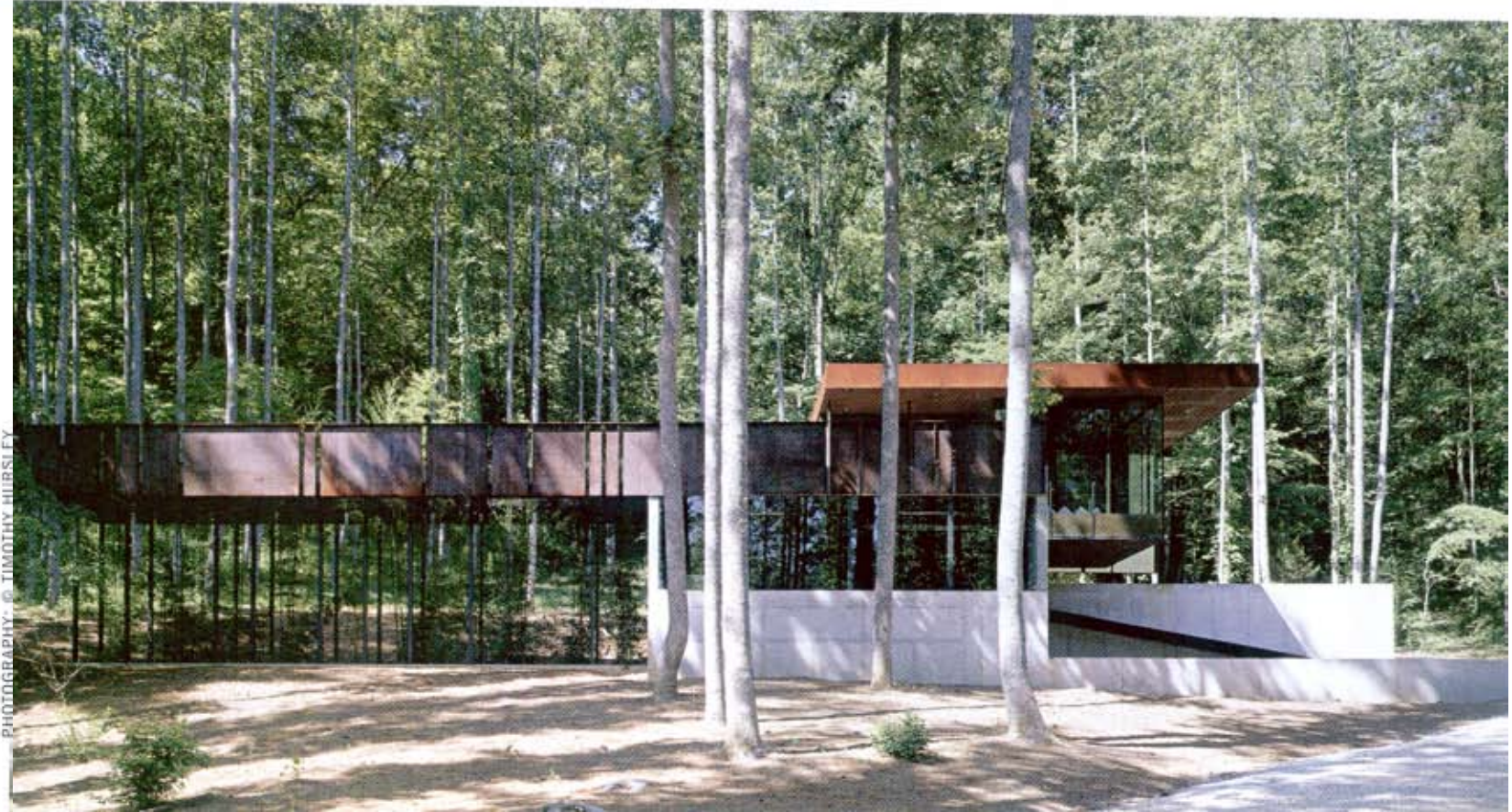
From both front (below) and back (above) elevations, the steel columns supporting the deck blend with the forest, mimicking the rhythm of poplar trees—as do the vertical slits in the Cor-ten parapet.
