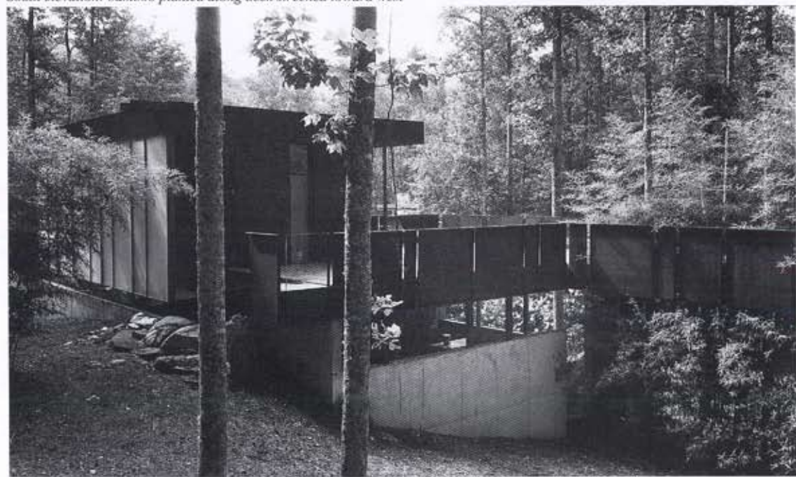
View from northwest: garage below deck having southwest corner window
