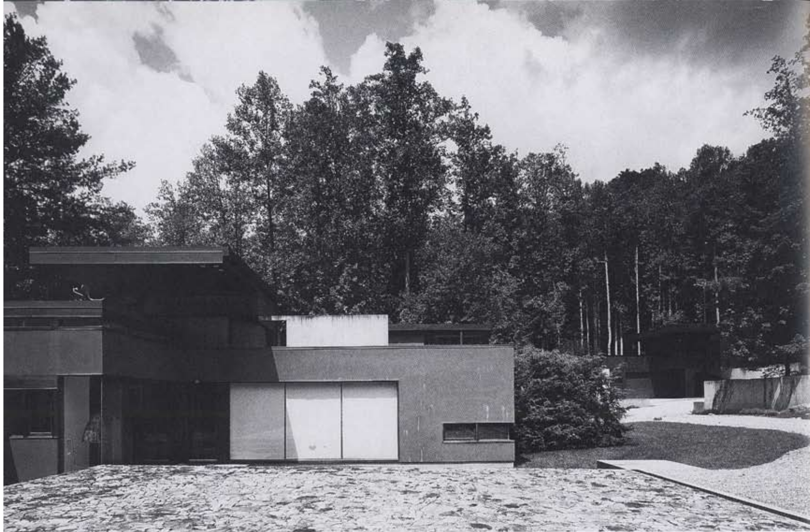
Main house(left) and new guest house(right)
