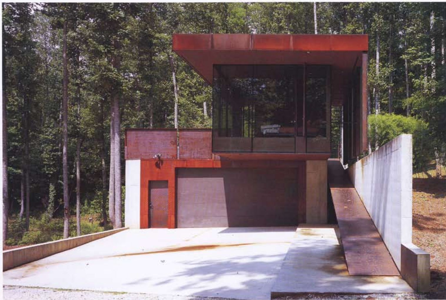
East view: ramp along concrete wall on north leading to deck on west
