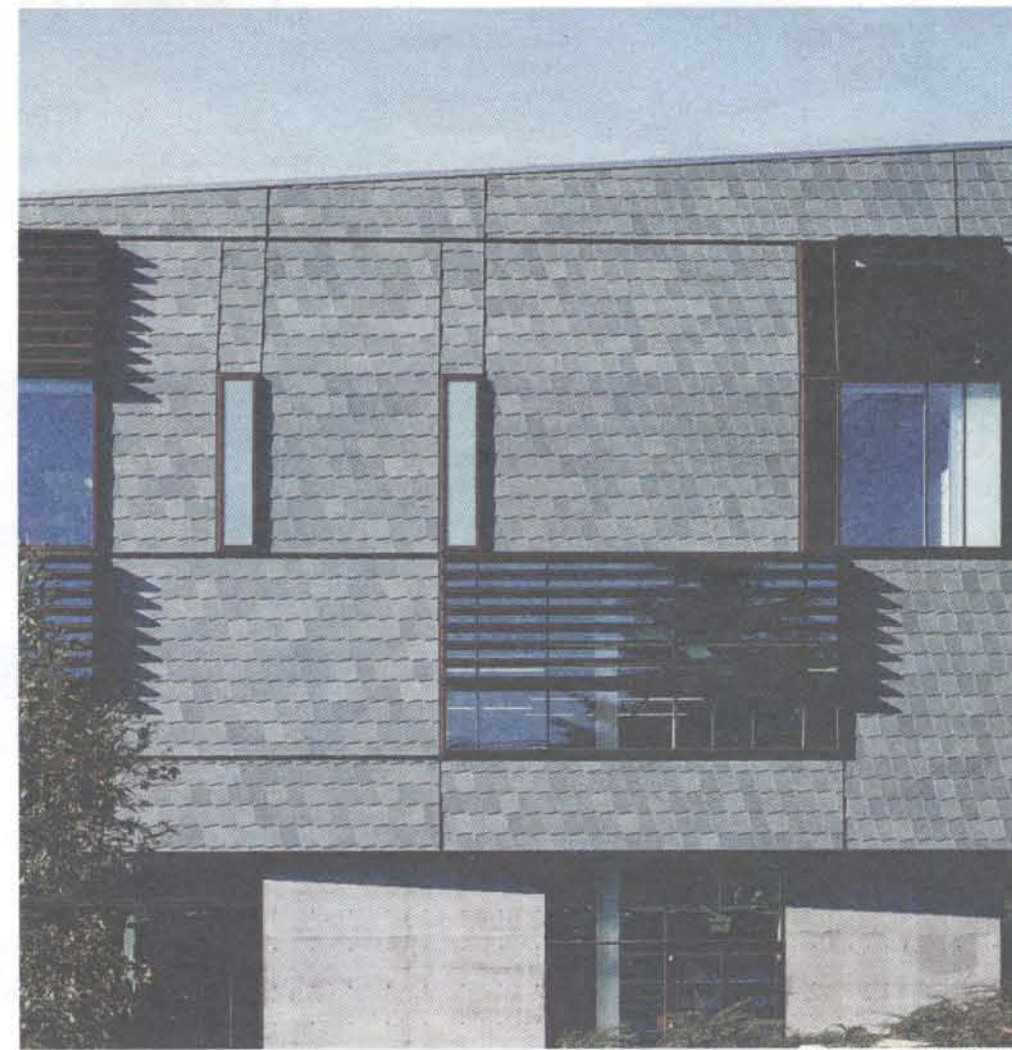
The music library's design has elements borrowed from nearby buildings in several different styles.
