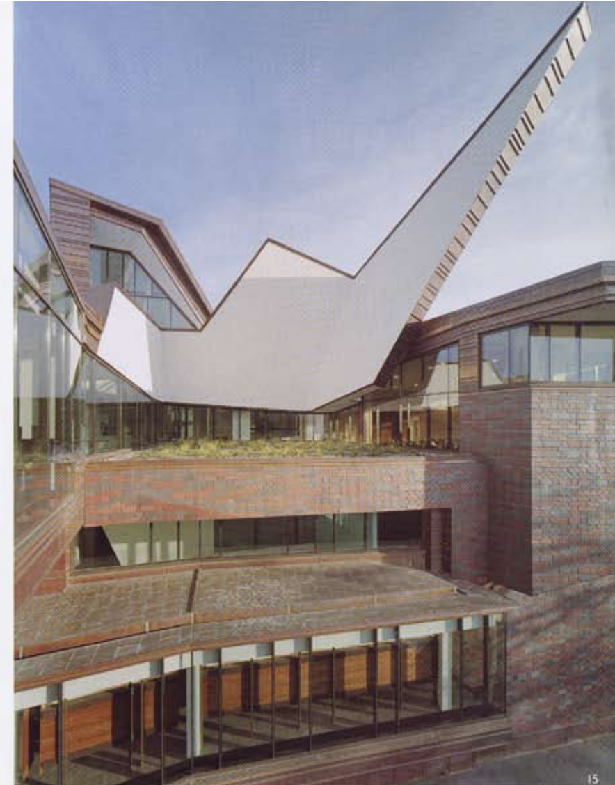
8. 微板楼 12. 东立面图 8. Mini Slab-building 12. East Elevation 9. 学院路层邮局内景 13. 南立面图 9. Interior of Post Office 13. South Elevation 10. 西立面图 14. 中央楼梯及采光井 10. West Elevation 14. Staircase and Light Well 11. A-A剖面图 15. 由水电厂西眺 11. Section A-A 15. View from the Physical Plant
