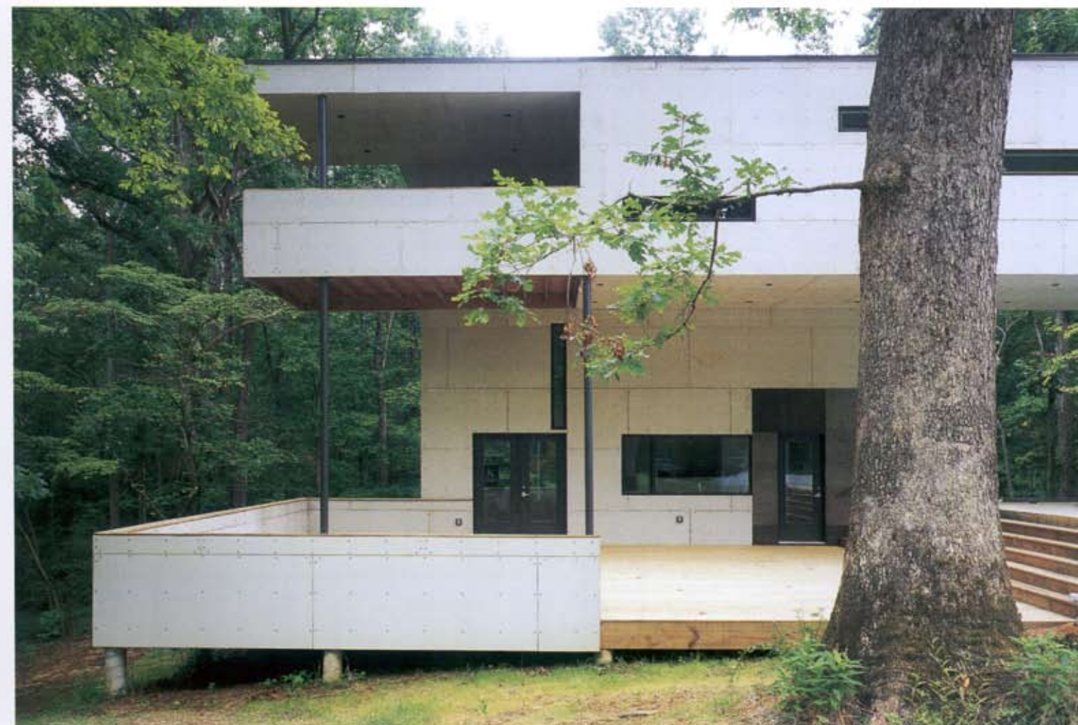
East elevation: deck of entrance
