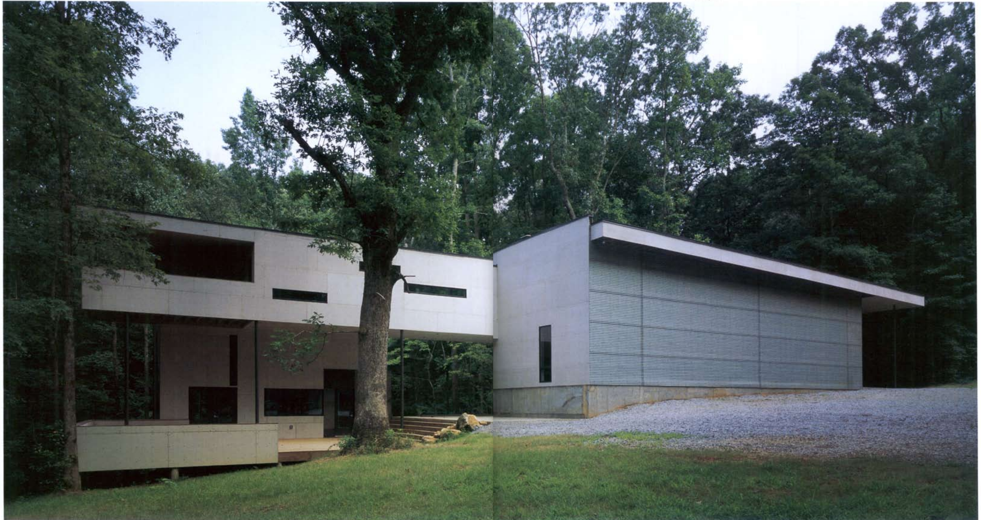
Overall view from south: studio wing on right
